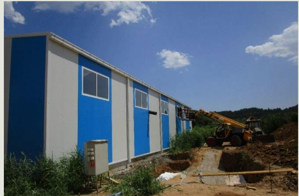
Delchevo – Water Treatment Plant
