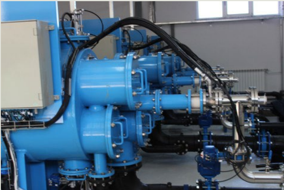
Gostivar Water Supply – Reservoir
