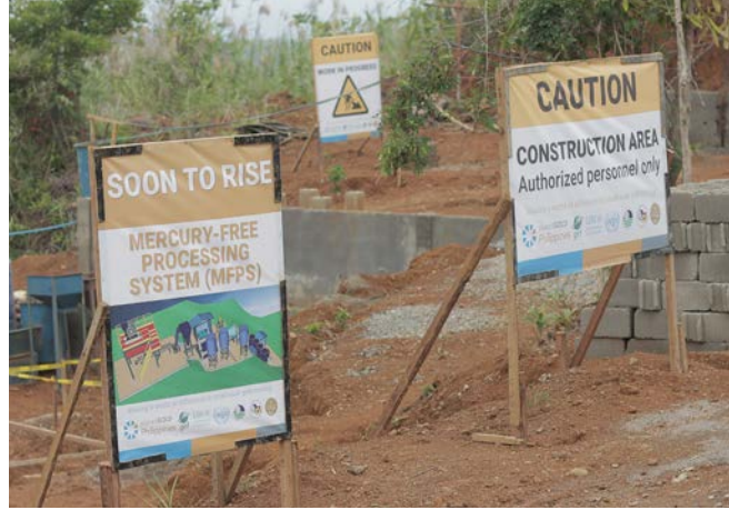
Signs marking the construction of a mercury-free processing system in Paracale
