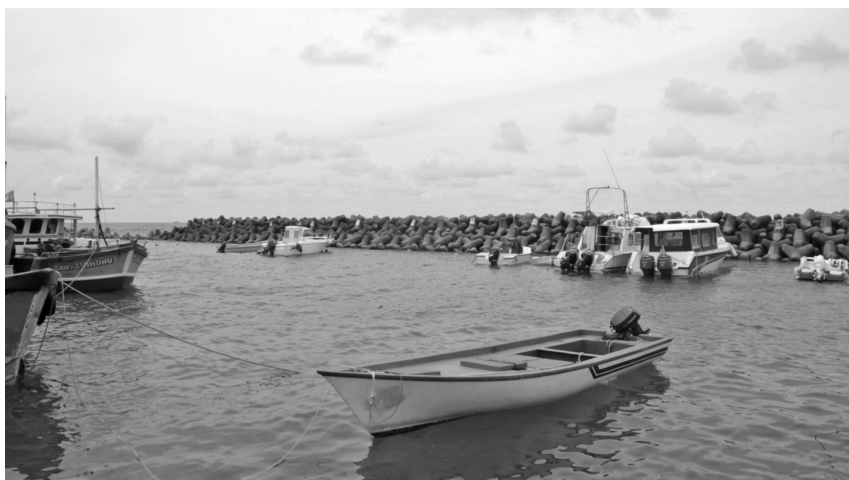
Figure 8.3 The $54 million tetrapod seawall surrounding Malé, Maldives
