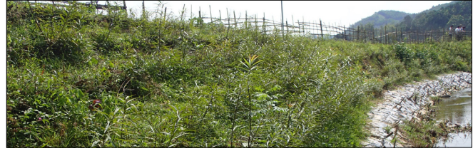
Overview of bioengineered riverbank protection in Bac Kan Province (September 2015) @ICEM
